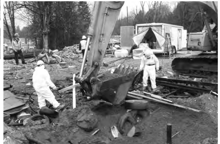
Workers removing asbestos contamination from the basement of the 'green garage'. Photos by David Munyak
