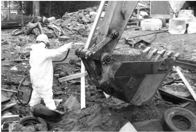
Workers removing asbestos contamination from the basement of the 'green garage'. Photos by David Munyak
